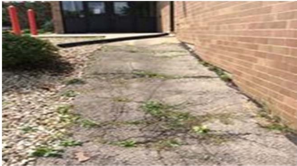
G3 - Cracked Asphalt
