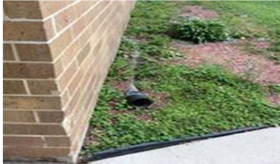
G4 – Damaged Drain Tile
