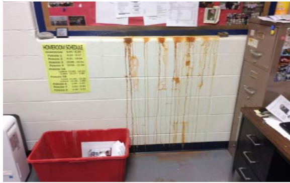
G16 – Exterior Wall Leaking
